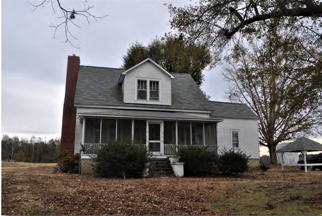
Figure 3.2: View of the primary (west) elevation of the Dunn-Scarborough-Frazier Farm (WA1788).
