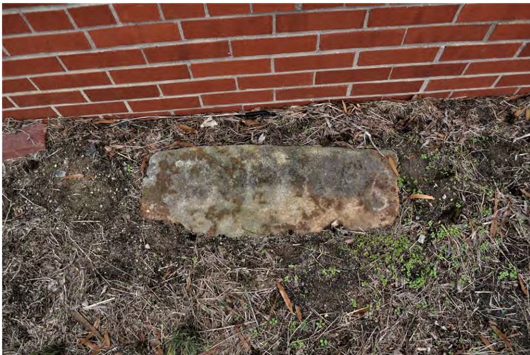
Figure 3.3: Date stone at base of 1940s chimney that reads “B.D. 1826.”
