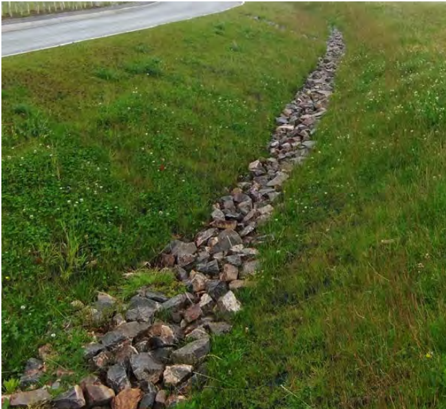
Figure 8: Typical vegetated swale conveyance system Source: https://salix-6aa7.kxcdn.com/wp-content/uploads/2014/09/7-VMax-P550-Vegetated-Swale-1024x768.jpg.webp
