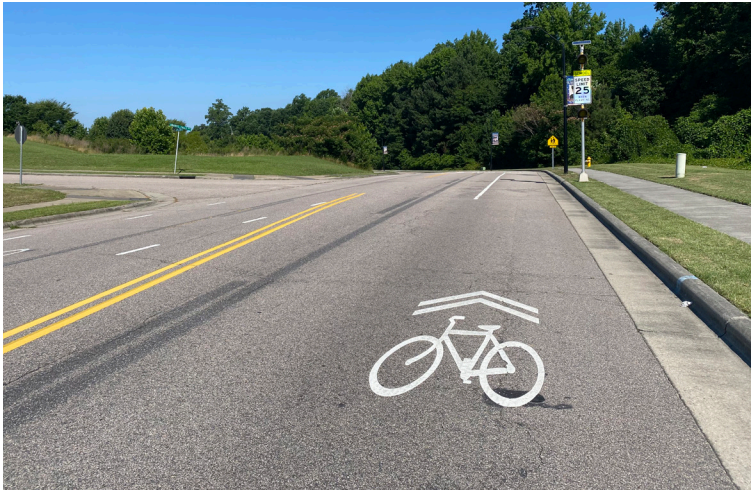
A shared lane marking at Granite Falls Blvd and W. Young St.
