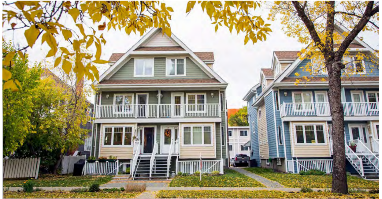
Figure 2-4: Multifamily housing does not have to be walk-ups or high rises. These apartments provide the aesthetics of a single family home while multiplying the potential density.
